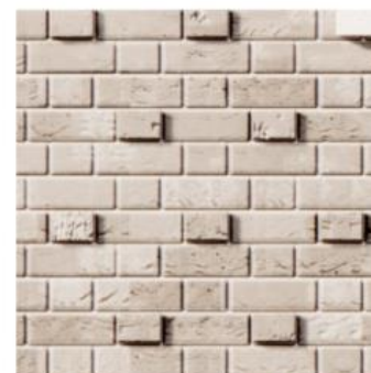
Flemish bond with alternating 25mm protruding header
