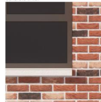
Feature colour framed windows with precast concrete sill.
