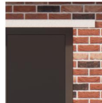
Dark framed windows with 75mm precast concrete lintel
